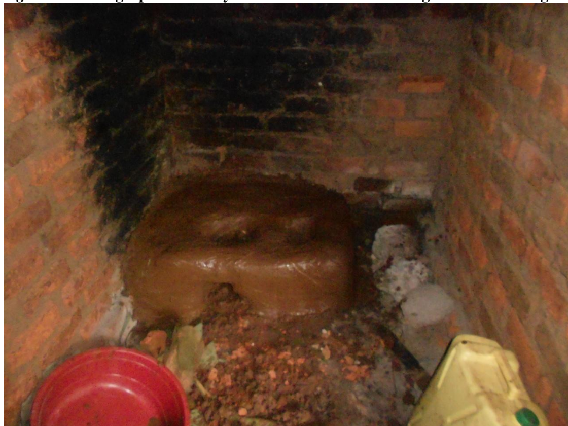
Figure 4: Photograph of a newly constructed domestic saving stoves in Katongero village-Kyebe S/C.
